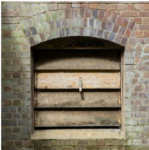
LV.01 Timber louvers/ Bespoke timber louvres to match the existing louvres
