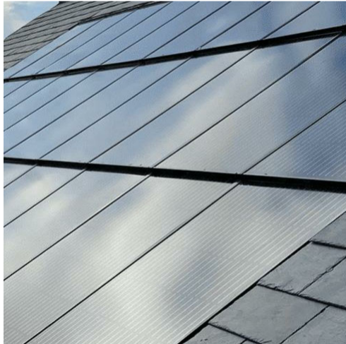
PV.01 Photo Voltaic Panels (Photovoltaic panels/ flush integrated photovoltaic panels
